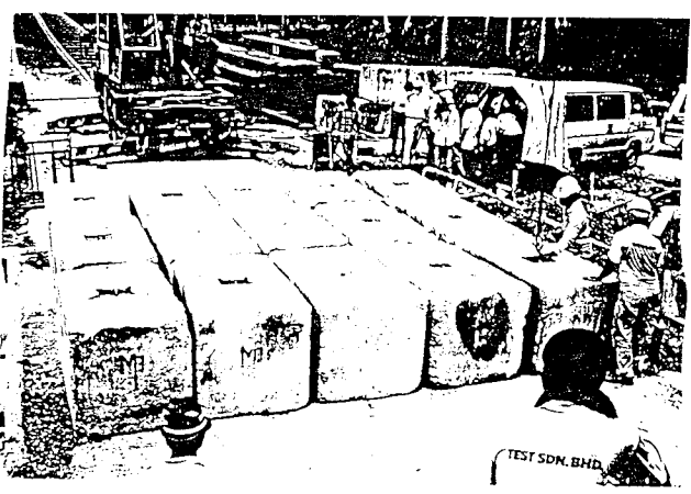
Figure 6: Scene of load test at 51.4 Tons
