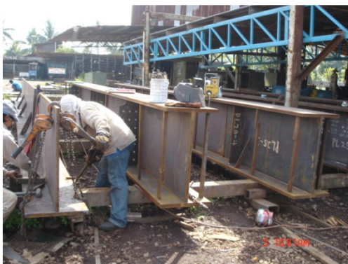
Fig. 8: Fabrication of the bridge
