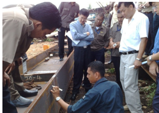
Fig. 9: Non-destructive testing witnessed by MPPP, JKR and the Consultant
