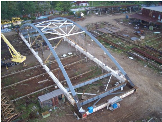
Fig. 10: Trial installation of the bridge at the fabrication yard
