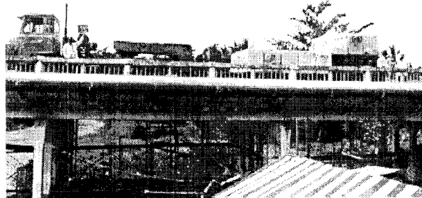
Figure 5: Load test on one of the spans with low loader at LL3
